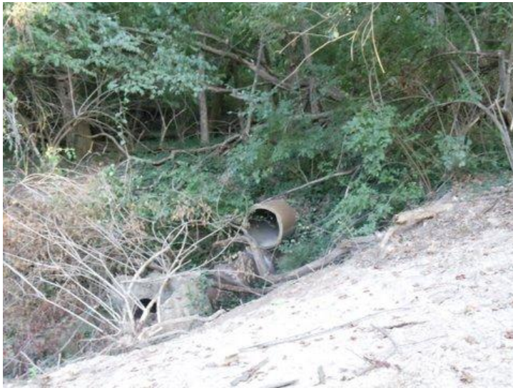
An older existing pipe that carries storm water from nearby subdivisions to the area
