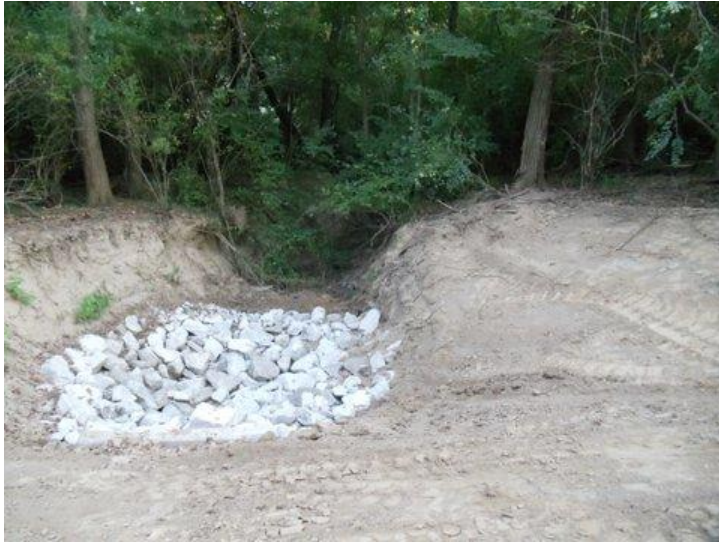
Large rocks placed in a storm water culvert to avoid erosion
